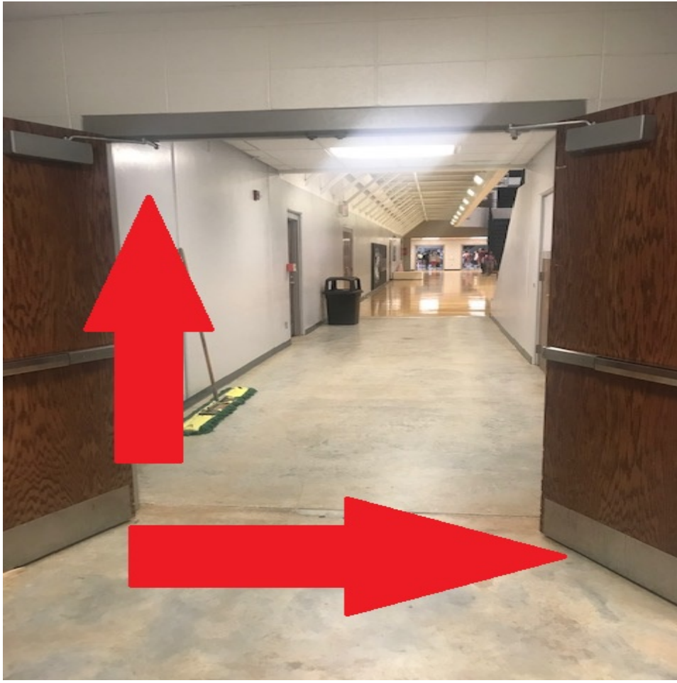
Entrance I: Performance Entrance to Main Gym—7' Tall; 5' 9" Wide.
