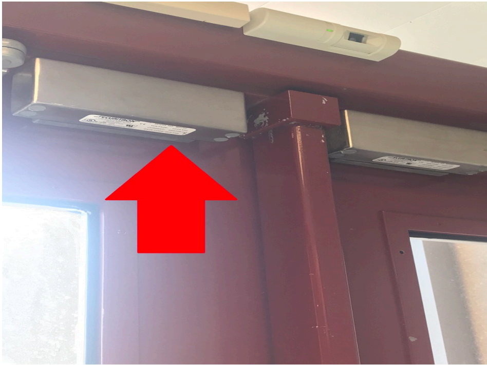
Entrance H: Prop Security Boxes on Outside Door. Measurements are figured with this included.
